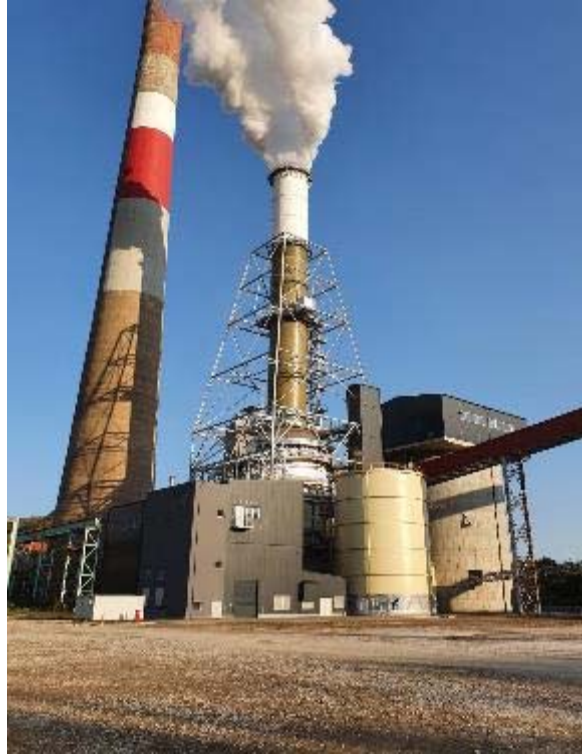
Figure 3-2: Overview of Ugljevik FGD plant
